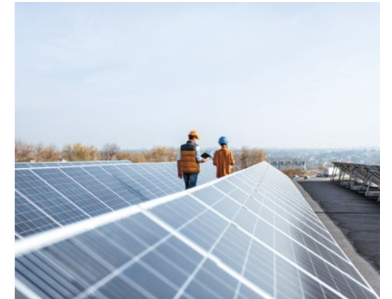
Future photovoltaic field in Lozère, France.
