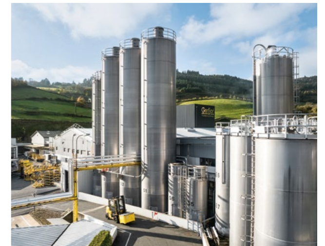
Modernised sites to reduce our energy consumption. Gerflor factory, Tarare, France.
